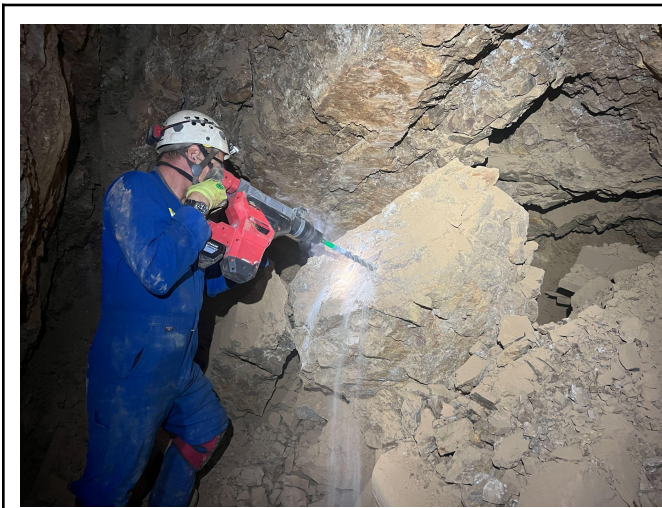
Figure 4: Drilling 1 ¼" holes for 1.4S blasting.
