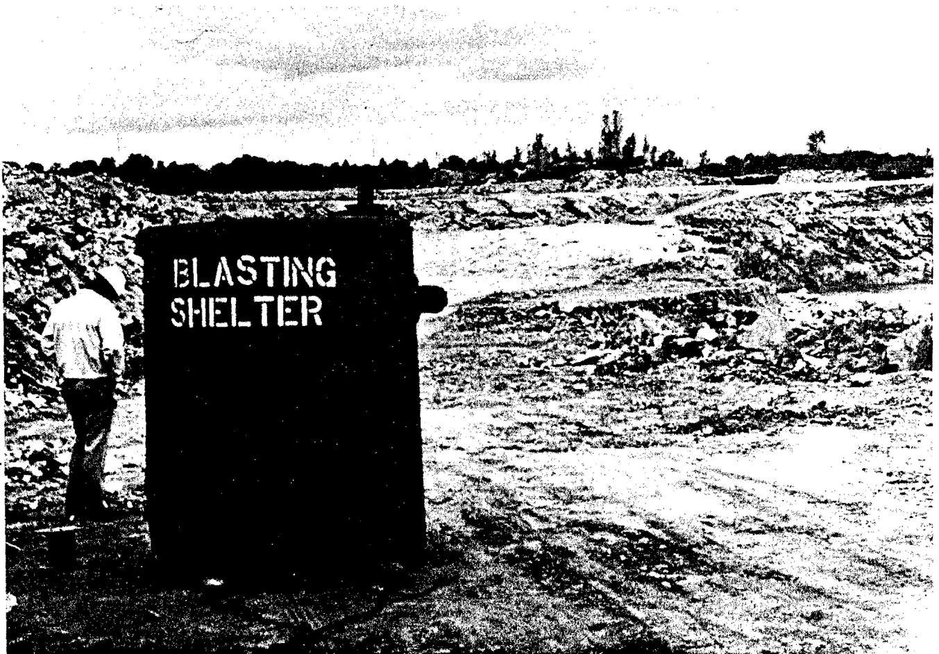
Figure 102.—Blasting shelter. (Courtesy Hercules Inc.)
