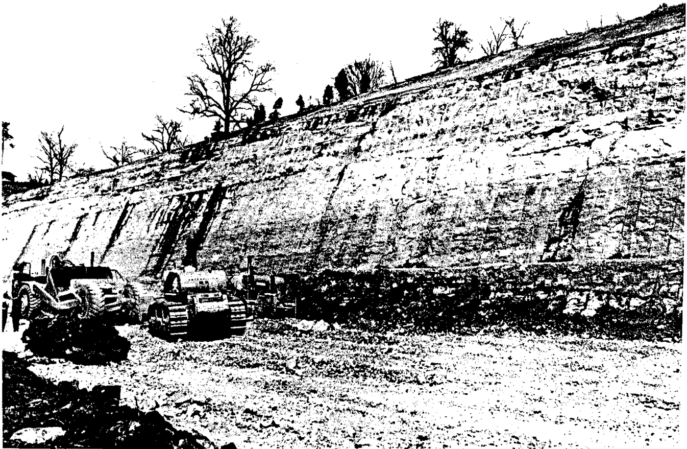
Figure 88.—Stable slope produced by controlled blasting. (Courtesy Austin Powder Co.)
