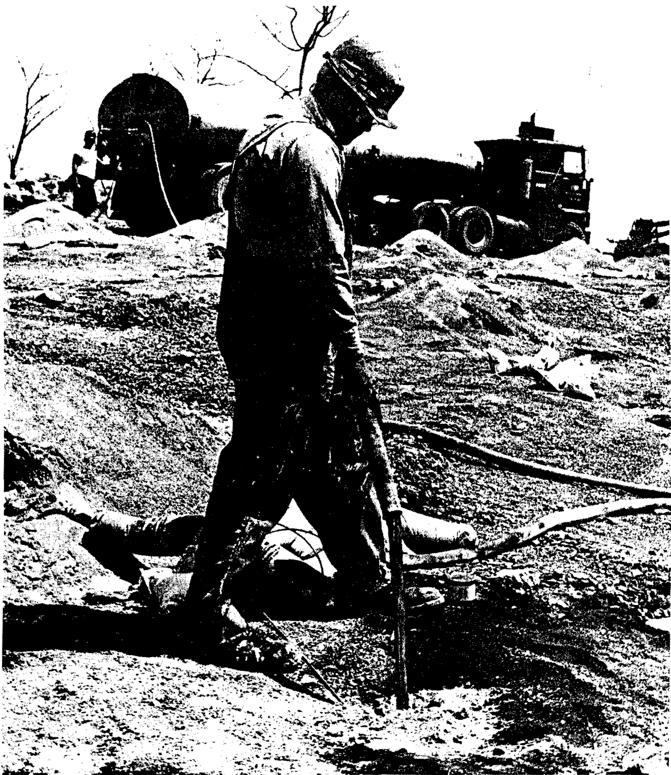
Figure 58.—Slurry leaving end of loading hose. (Courtesy Du Pont Co.)
