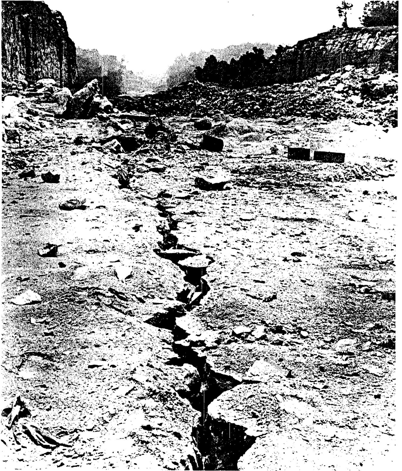
Figure 89.—Crack generated by a presplit blast. (Courtesy Austin Powder Co.)
