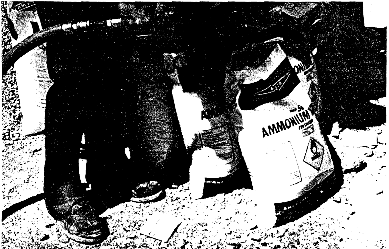
Figure 16.—Field mixing of AN-FO. (Courtesy Hercules Inc.)
