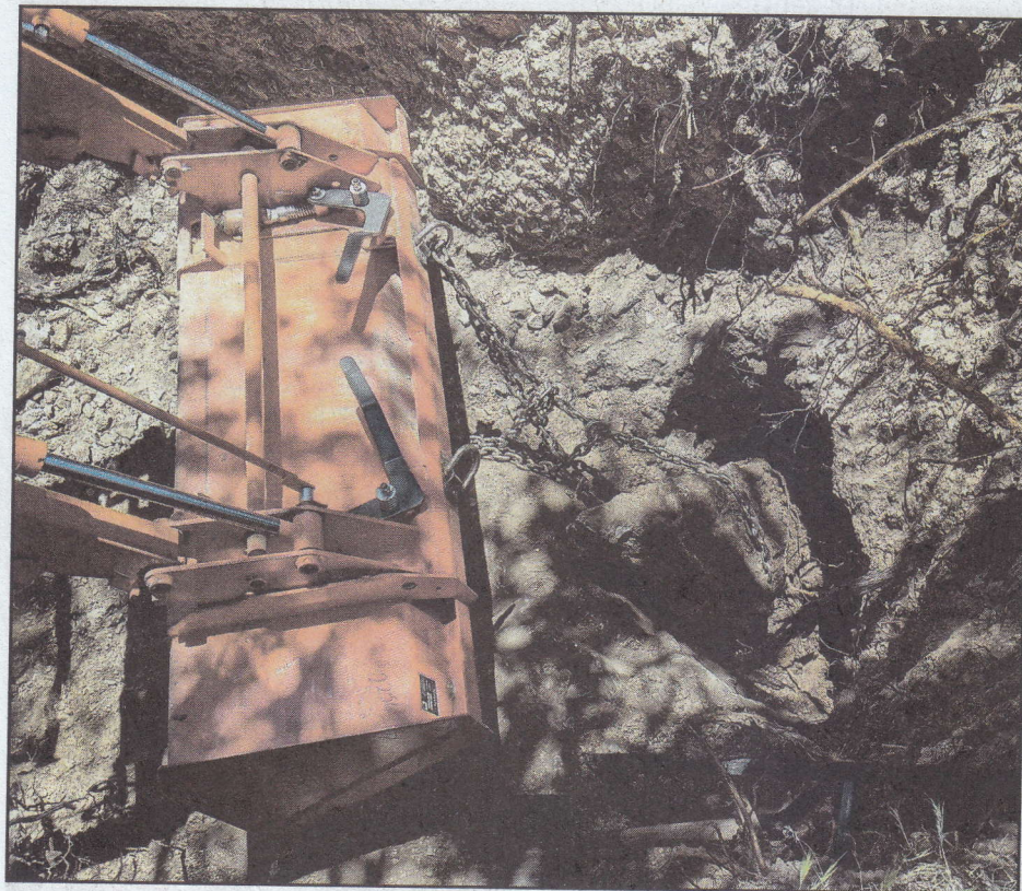
Sometimes big boulders can be slung with a heavy chain and dragged out of the hole they are in without further breaking.
