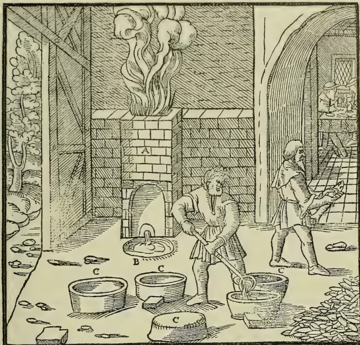
A—FURNACE. B—FOREHEARTH. C—OBLONG MOULDS.
