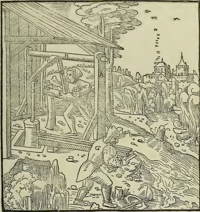
A—POSTS. B—AXLE. C—WOODEN BARS. D—PISTON ROD. E—SHORT PIECE OF WOOD. F—DRAIN. G—THIS MAN IS DIVERTING THE WATER WHICH IS FLOWING OUT OF THE DRAIN, TO PREVENT IT FROM FLOWING INTO THE TRENCHES WHICH ARE BEING DUG.
