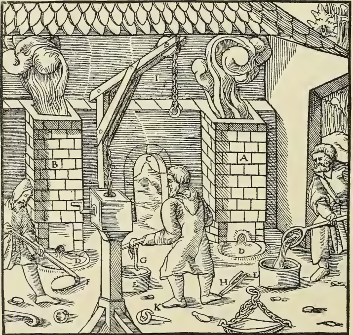
A—FURNACE IN WHICH "SLAGS" ARE RE-SMELTED. B—FURNACE IN WHICH COPPER IS ALLOYED WITH LEAD. C—DOOR. D—FORE-HEARTHES ON THE GROUND. E—COPPER MOULDS. F—RABBLE. G—HOOK. H—CLEFT STICK. I—ARM OF THE CRANE. K—THE HOOK OF ITS CHAIN.
