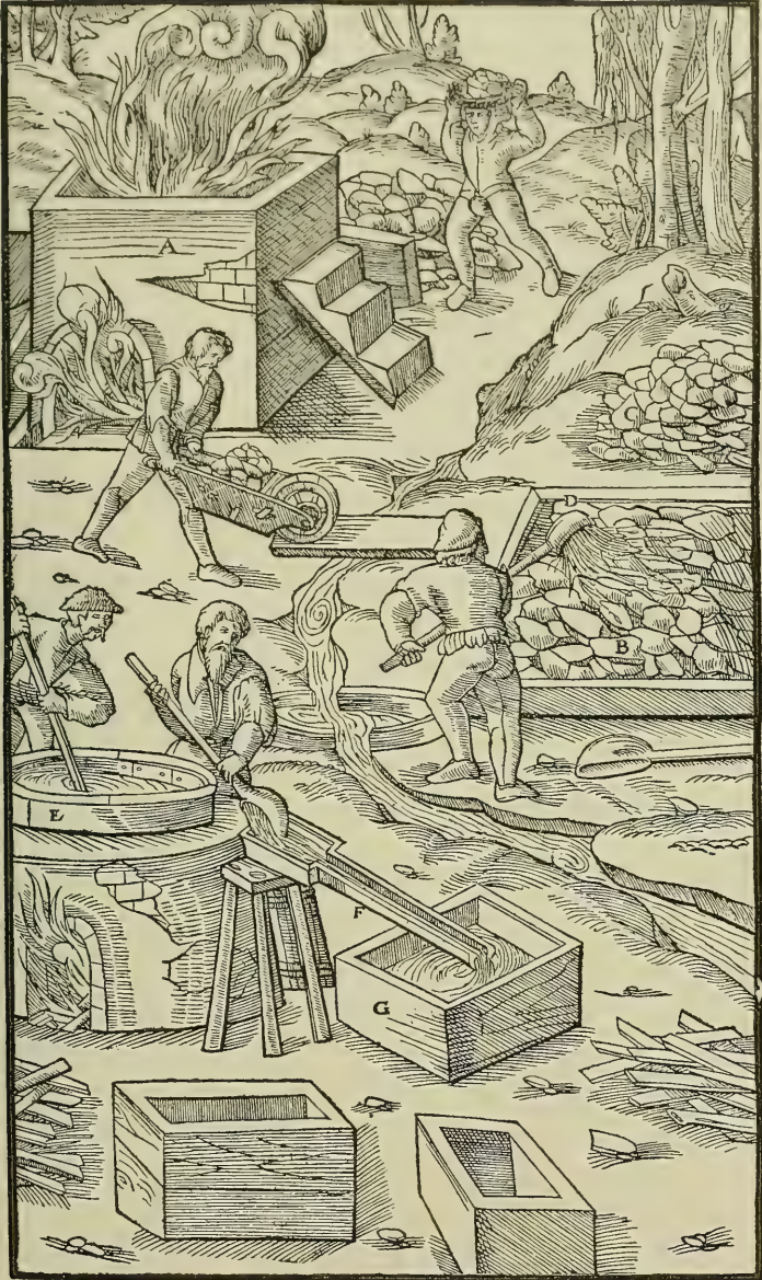
A—FURNACE. B—ENCLOSED SPACE. C—ALUMINOUS ROCK. D—DEEP LADLE. E—CALDRON. F—LAUNDER. G—TROUGH.
