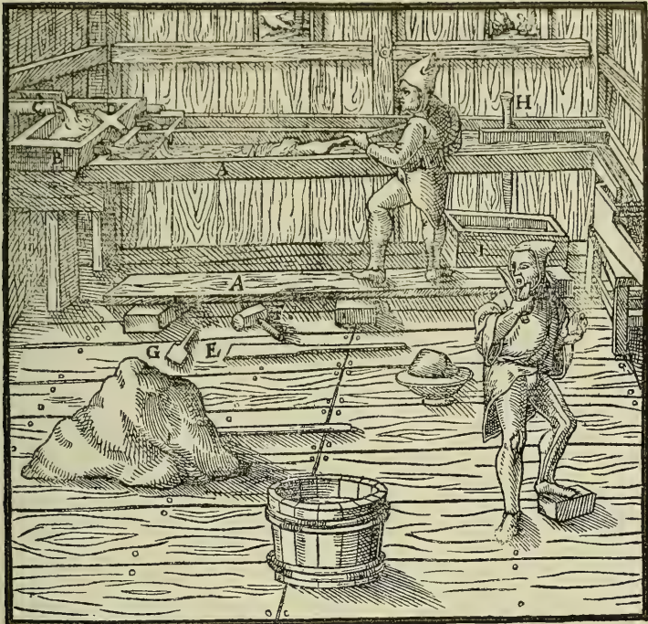
A—STRAKES. B—TANK. C—LAUNDER. D—PLUG. E—WOODEN SHOVEL. F—WOODEN MALLET. G—WOODEN SHOVEL WITH SHORT HANDLE. H—THE PLUG IN THE STRAKE. I—TANK PLACED UNDER THE PLUG.
