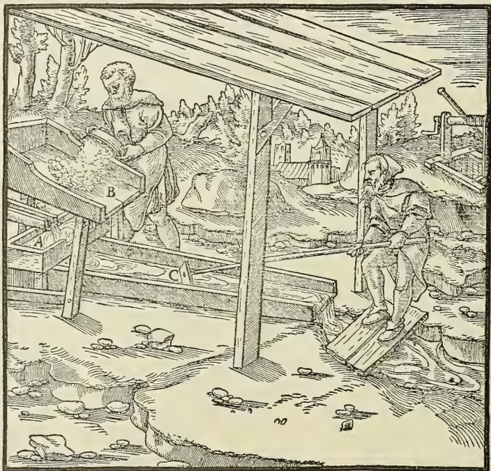
A—TROUGH. B—PLATFORM. C—WOODEN SCRUBBER.
