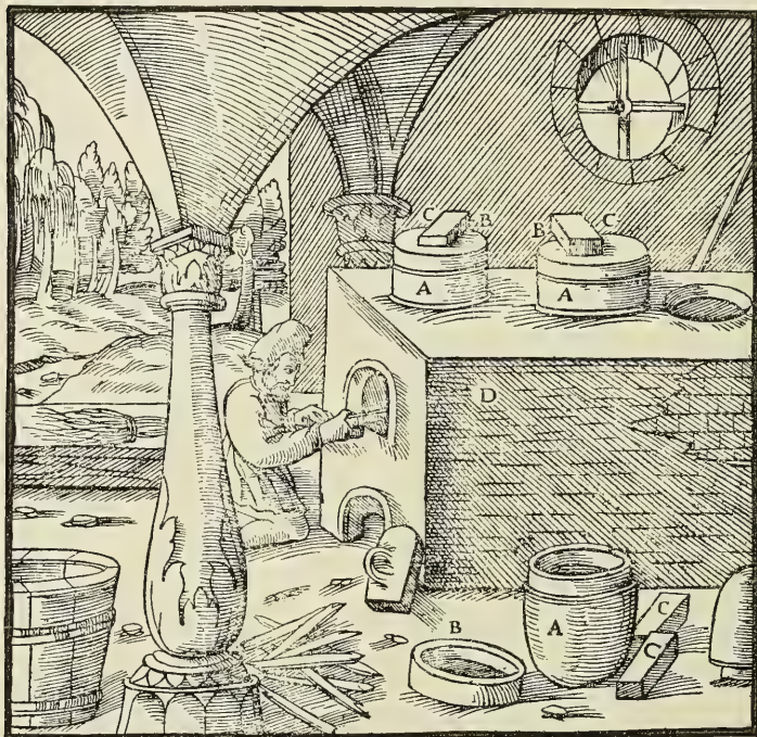
A—POTS. B—LIDS. C—STONES. D—FURNACE.
