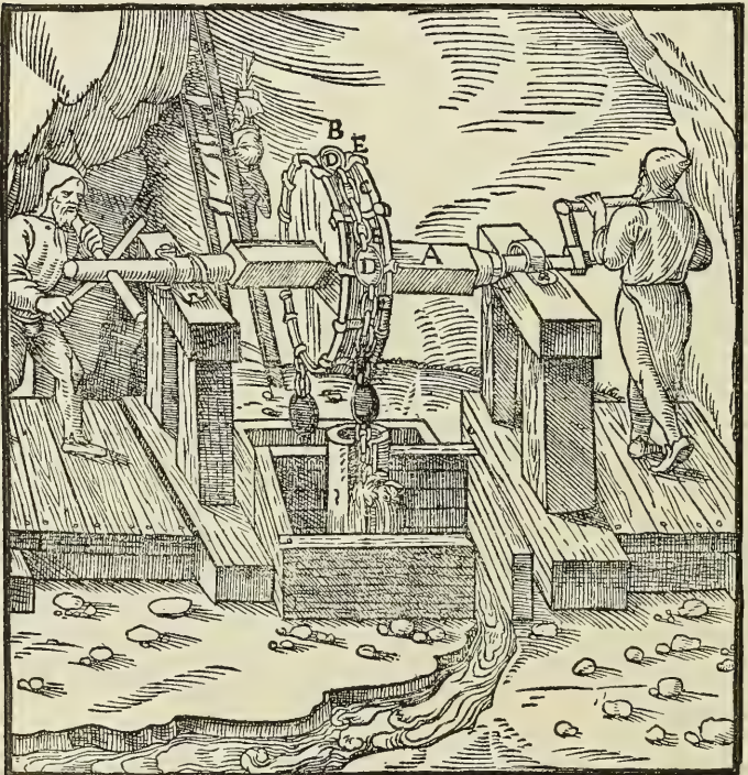
A—AXLE. B—DRUM. C—DRAWING-CHAIN. D—BALLS. E—CLAMPS.
