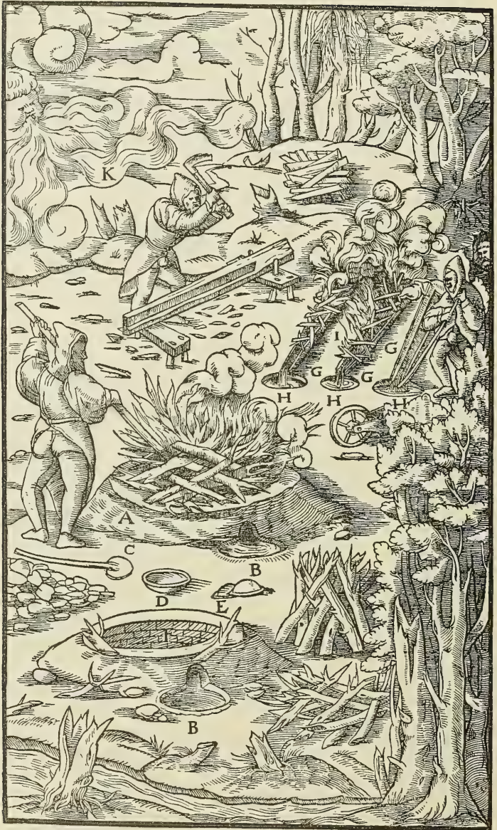
A—PIT ACROSS WHICH WOOD IS PLACED. B—FOREHEARTH. C—LADLE. D—IRON MOULD. E—CAKES. F—EMPTY POT LINED WITH STONES IN LAYERS. G—TROUGH. H—PITS DUG AT THE FOOT OF THE TROUGH. I—SMALL WOOD LAID OVER THE TROUGH. K—WIND.
